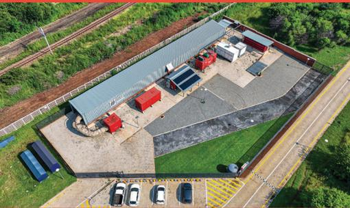
Aerial view of the H<sub>2</sub> piloting cluster and the dedicated PV installation (70kWp, combined) at the NWU HySA Infrastructure facilities to supply **renewable energy (RE)** for green hydrogen production.
