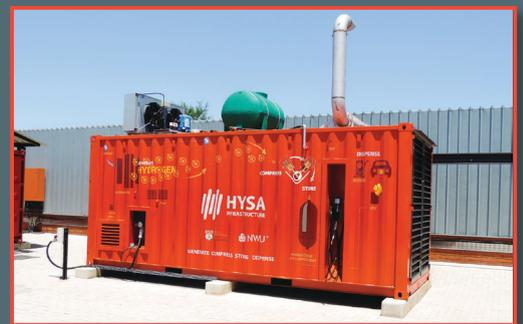
Above are some key elements of the “green” H<sub>2</sub> piloting cluster at NWU HySA Infrastructure facilities, including 350 bar H<sub>2</sub> mobile refuelling system, PEM 6 Nm<sup>3</sup>/h H<sub>2</sub> electrolyser, H<sub>2</sub> storage via Liquid Organic Hydrogen Carrier technology (LOHC) with energy storage capacity equivalent of 1 MWh and 13500 L of compressed H<sub>2</sub> storage.
